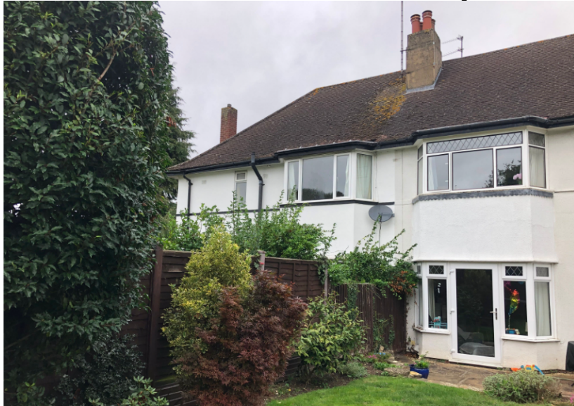
Rear of application property and the adjoining property to the west
