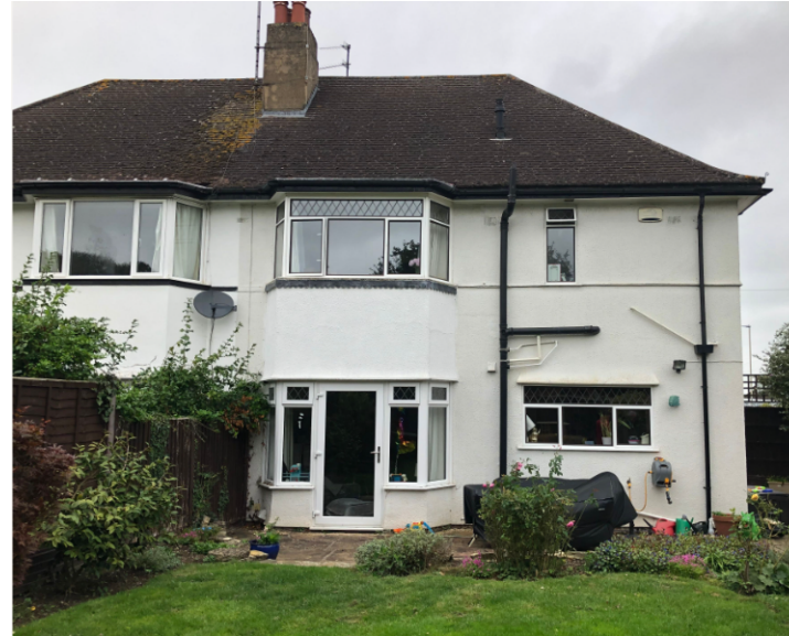
Rear of application property
